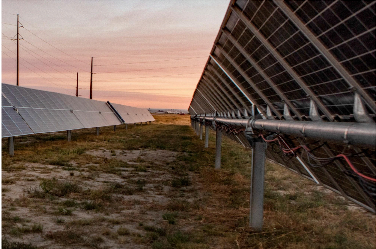
Solar farm in California. Source: Adobe Stock.
